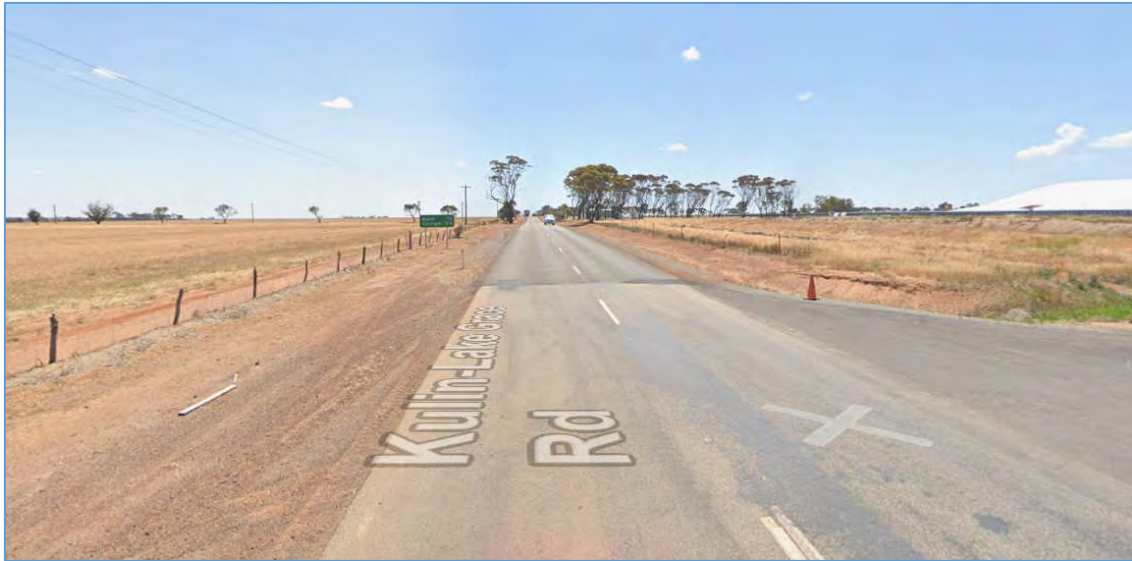
Figure 14: Kulin-Lake Grace Road / CBH Site Exit Intersection Looking North
