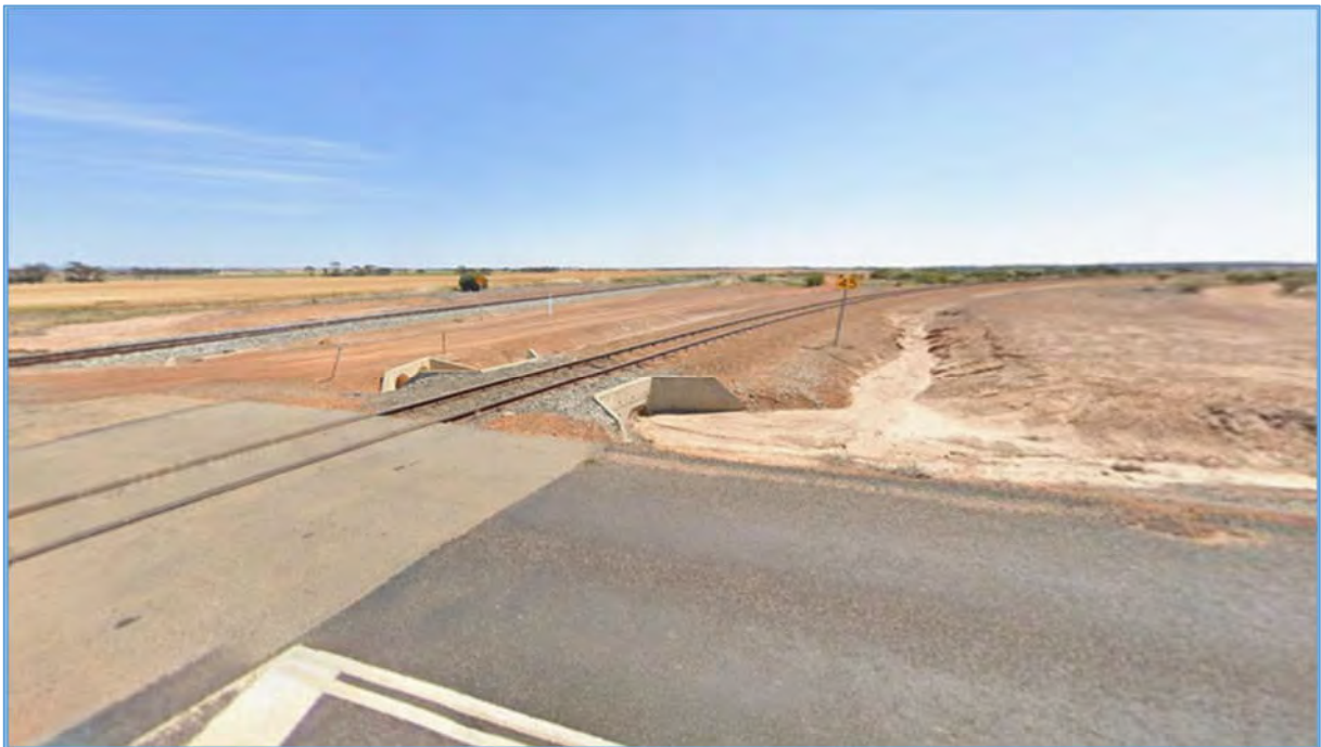
Figure 43: Biddy-Camm Level Crossing - East Side Looking North
