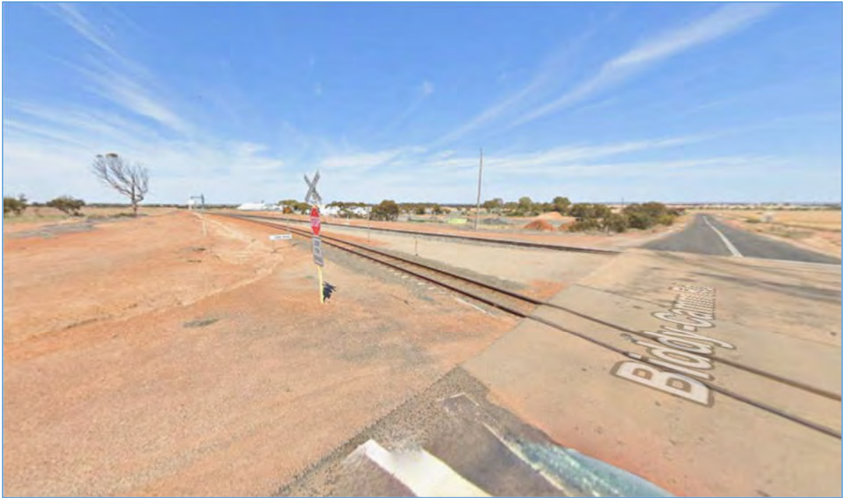
Figure 44: Biddy-Camm Level Crossing - East Side Looking South
