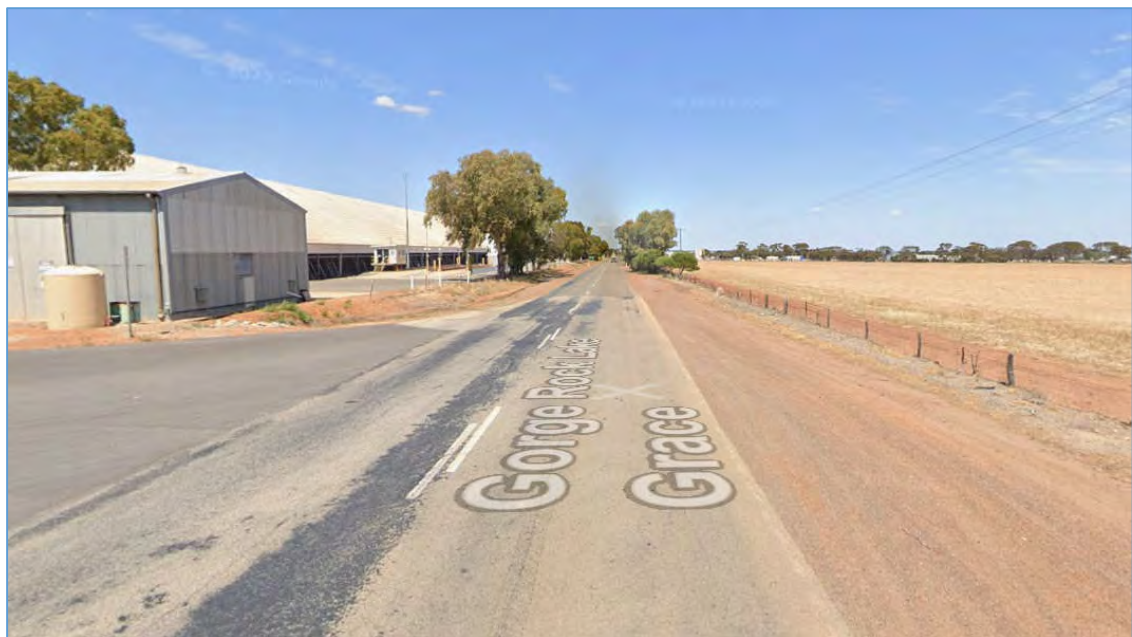
Figure 15: Kulin-Lake Grace Road / CBH Site Exit Intersection Looking South
