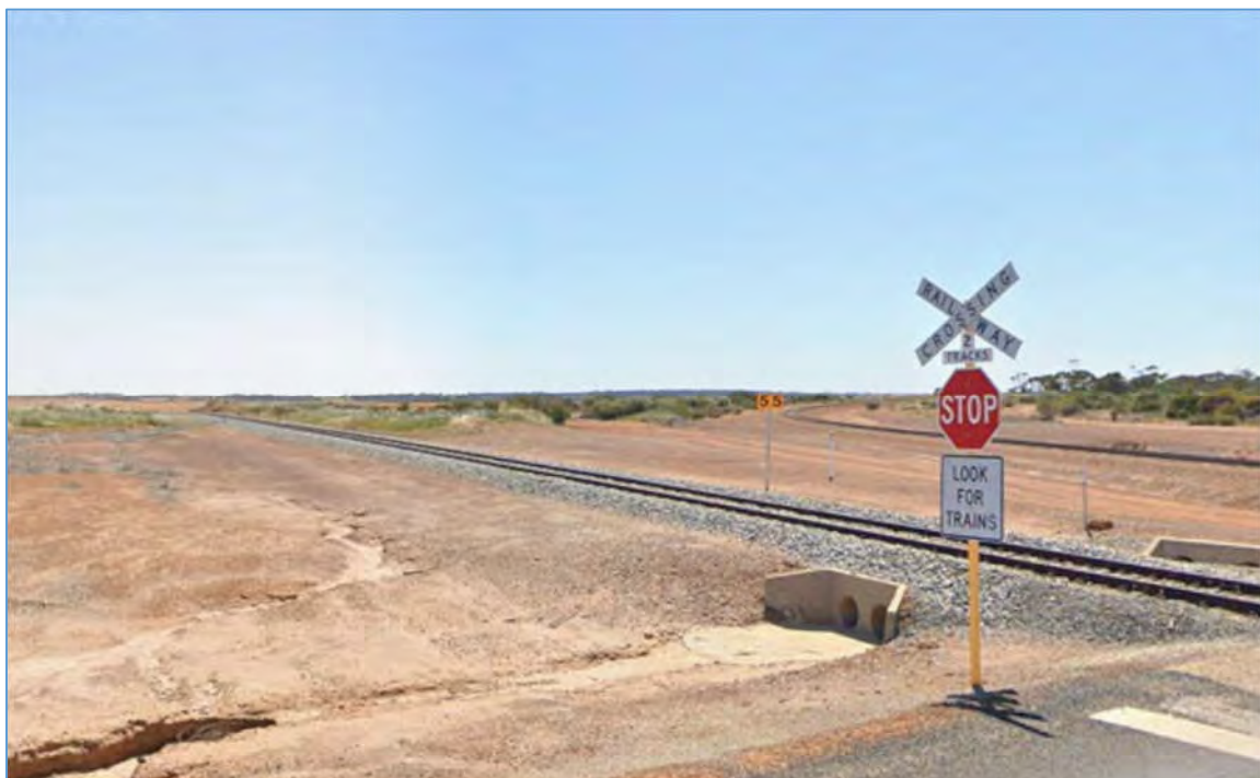
Figure 41: Biddy-Camm Level Crossing - West Side Looking North
