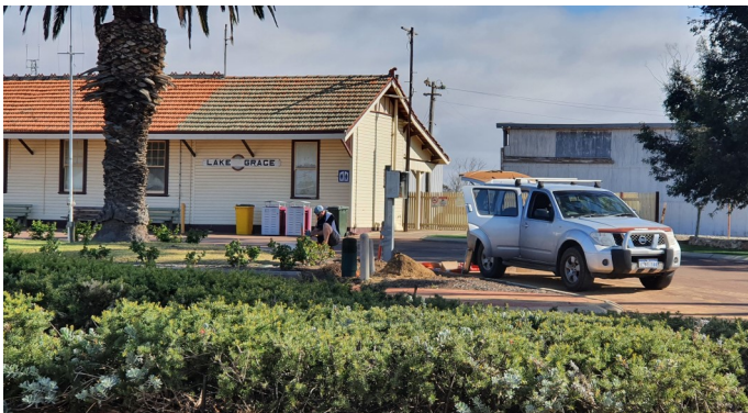
New fast car charger installed
