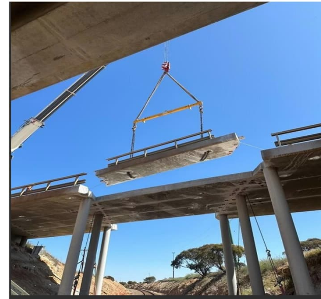
Bridge 629 on Great Eastern Highway
