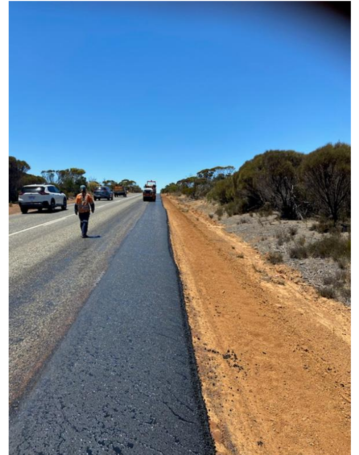
Asphalt widening Collie – Lake King
