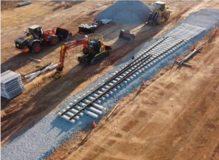
Brookton rail siding extension
