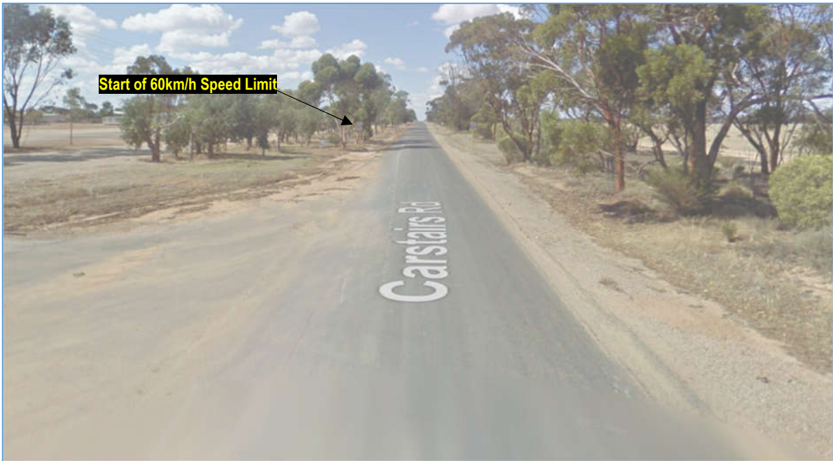
Figure 18: Southern CBH Lake Varley Site Exit / Carstairs Road - Looking East
