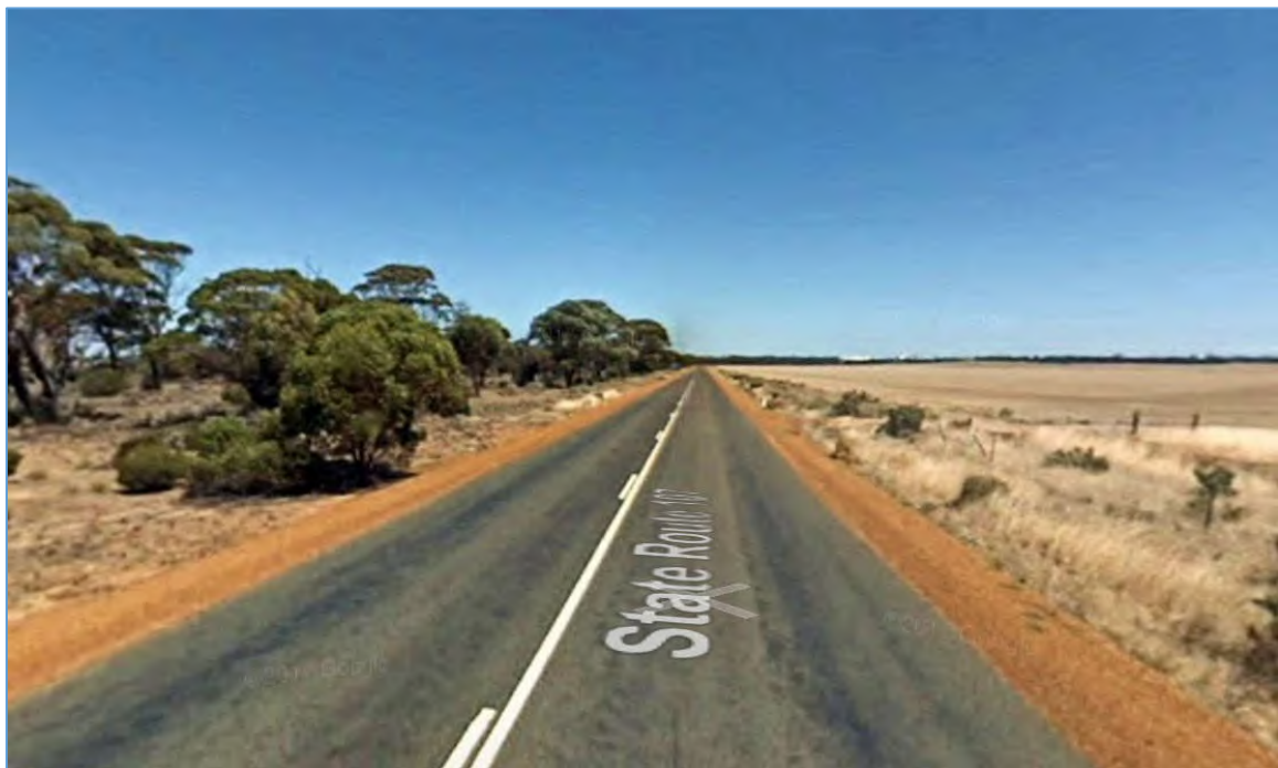
Figure 13: SISD Looking West
